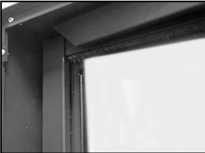
Figure 58: Installing top trim.
